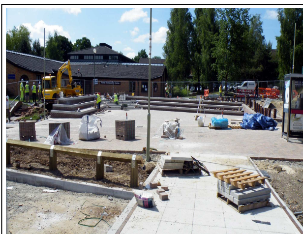
Forest Centre Integration Project – Whitehill & Bordon
