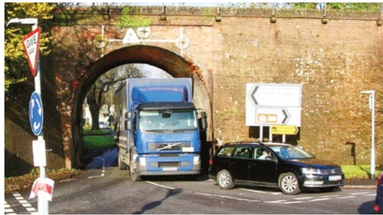
Butts Bridge – a brick arch structure.
