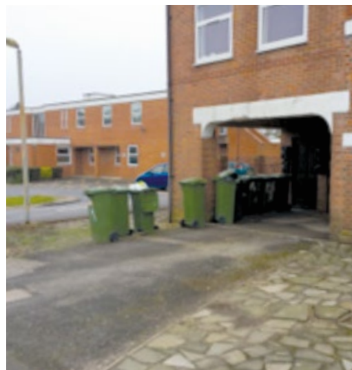
Waste Bin Storage at Anstey Road, Alton
