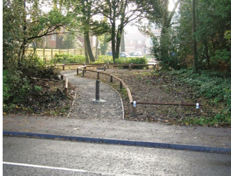
Footpaths can provide attractive links for pedestrians.
