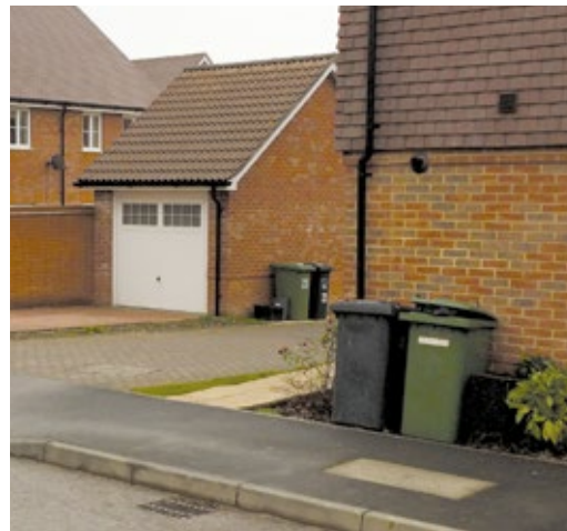
Waste Bin Storage at Barley Field Estate, Alton
