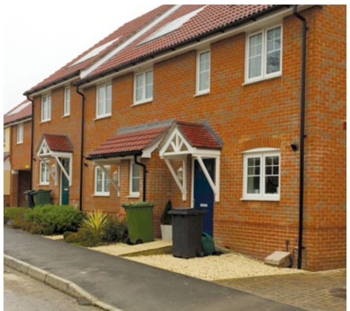
Waste Bin Storage at Barley Field Estate, Alton
