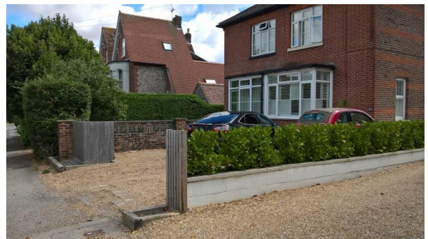
Figure 20.8 Frontage opened up for vehicle access
