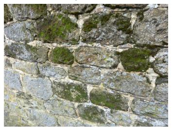
Irregular mortar joints in a boundary wall with fragments of galetting
