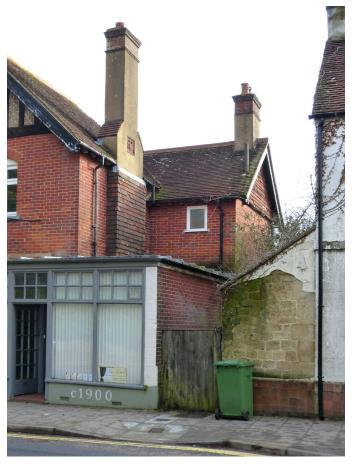
A section of exposed masonry wall behind failing render
