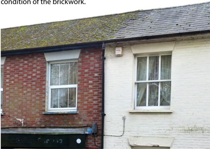
*18th- or early 19th-century brickwork, which has been left exposed at one address and painted over next door*
