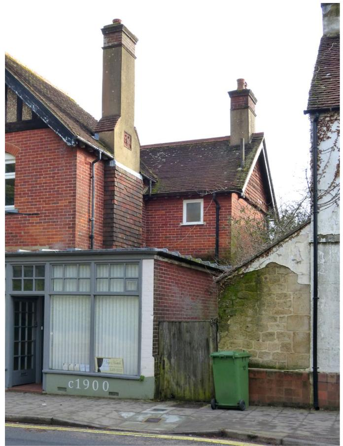
*A section of exposed masonry wall behind failing render*
