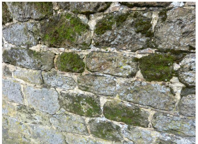
*Irregular mortar joints in a boundary wall with fragments of galetting*
