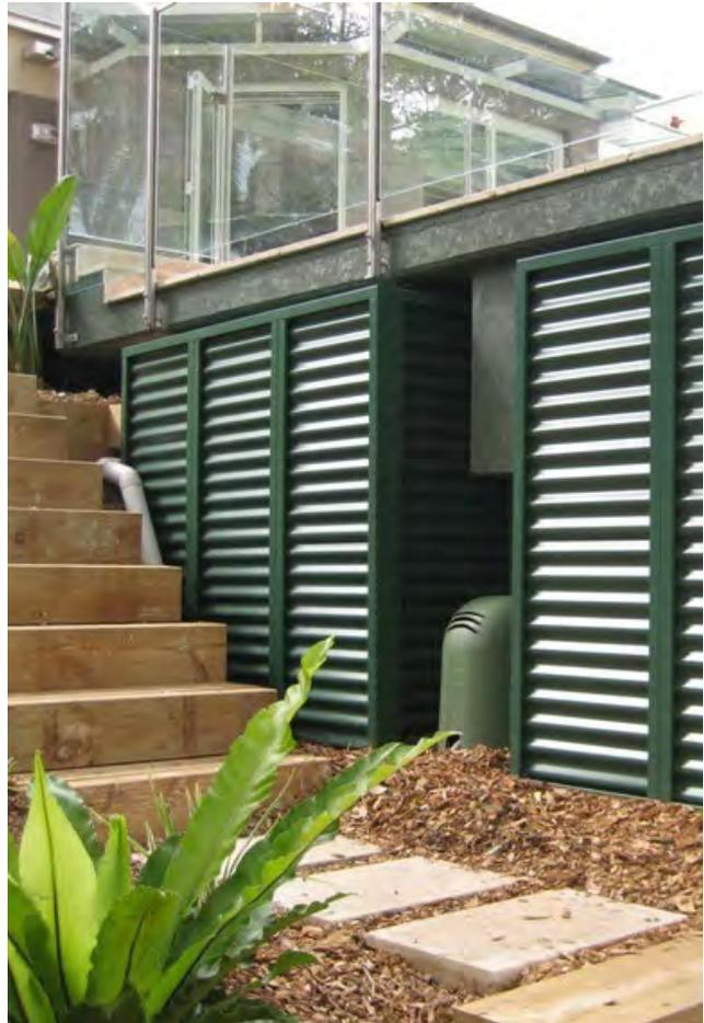
Figure 109: Example of a modular water tank.
