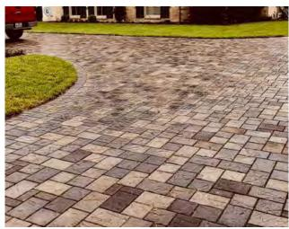
**Figure 111:** A good example of permeable paver (Source: https://www.paverconnection.com/testimonial/hedwig-village-permeable-driveway-and-patio-upgrade/)
