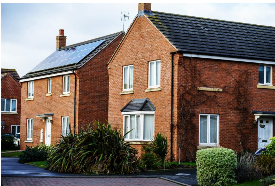
Figure 1. Example of roof-mounted solar PV panels.
