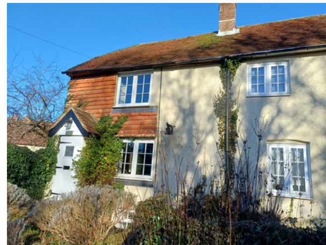
Climbing plants such as ivy have the potential to disturb and displace historic fabric. Vegetation growing around downpipes can indicate the presence of moisture caused by leaks or blockages.
