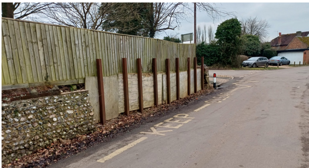
This temporary repair to a missing section of flint boundary wall on Church Street detracts from the character of the streetscape and provides an opportunity for enhancement.
