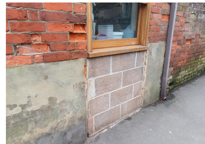
The incorporation of modern breeze blocks with a highly visible elevation on this historic building is detrimental to the historic character of the building and the wider conservation area.
