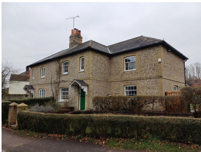
Knapped flint, yellow brick and flint used in combination at 13-15 Finchdean Road.
