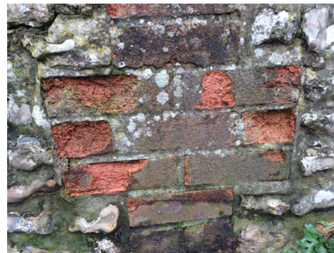
This section of boundary wall has been subject to inappropriate repairs with cement-based mortar. As moisture cannot escape through the mortar, it instead moves through the bricks, causing them to degrade over time. Failed pointing has not been replaced, leaving large gaps in the wall where plants can take root.
