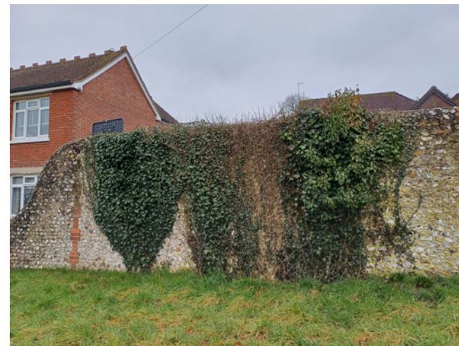
Heavy vegetation growth to the flint boundary wall enclosing the grounds of Deerleap. If left unmanaged, vegetation can displace historic fabric and encourage moisture ingress.
