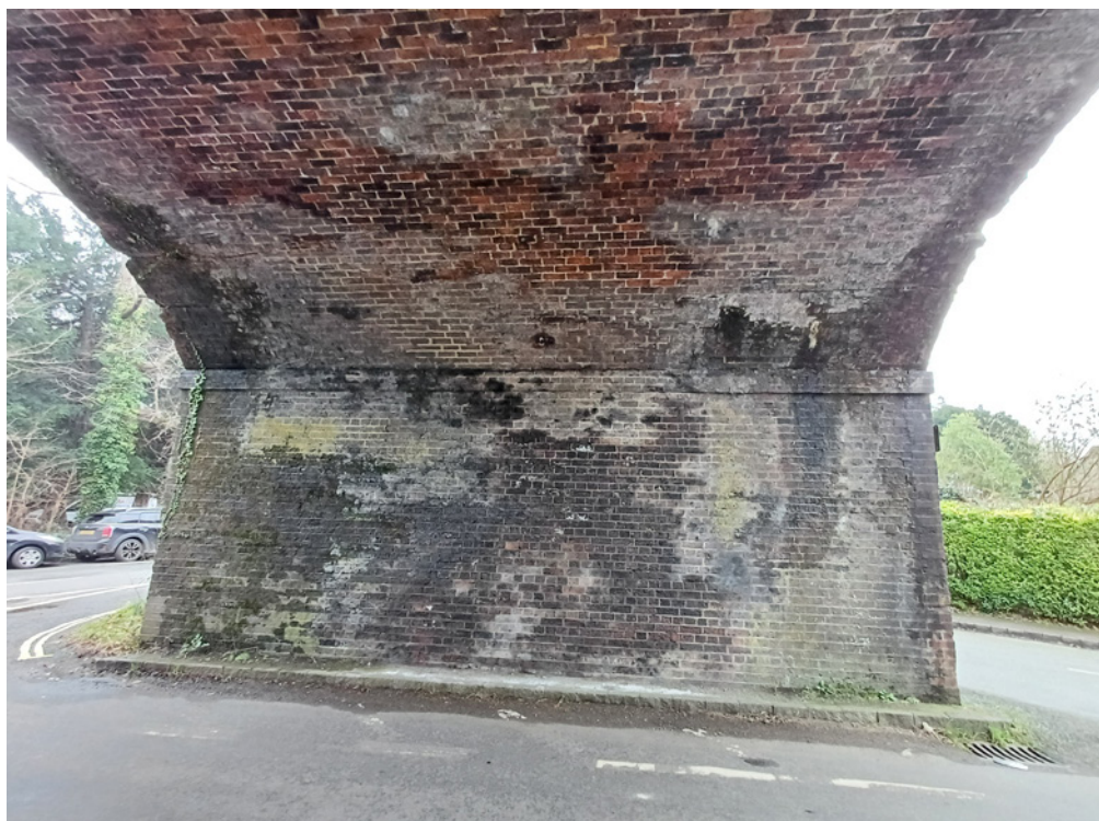
Heavy efflorescence (salt deposits) and staining to the railway bridge.
