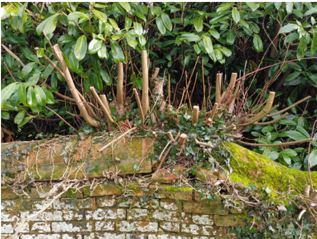
When left unmanaged, vegetation can take root in historic joints and push fabric out of place as it grows.
