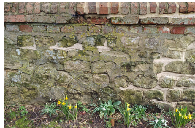
This section of malmstone boundary wall off Ryebidge Lane has been subject to inappropriate repairs with cement-based mortar. As moisture cannot escape through the mortar, it instead moves through the masonry, causing it to degrade over time.
