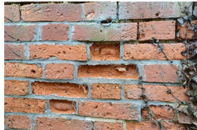
A section of boundary wall to the Old Dairy off Ryebidge Lane. This illustrates the damage caused to fabric through the use of cementitious mortar to re-point historic brickwork.
