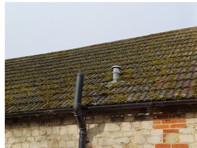
The uPVC downpipe and interlocking concrete roof tiles to this historic agricultural structure at West End Farm detracts from the historic character of the building and the wider conservation area.
