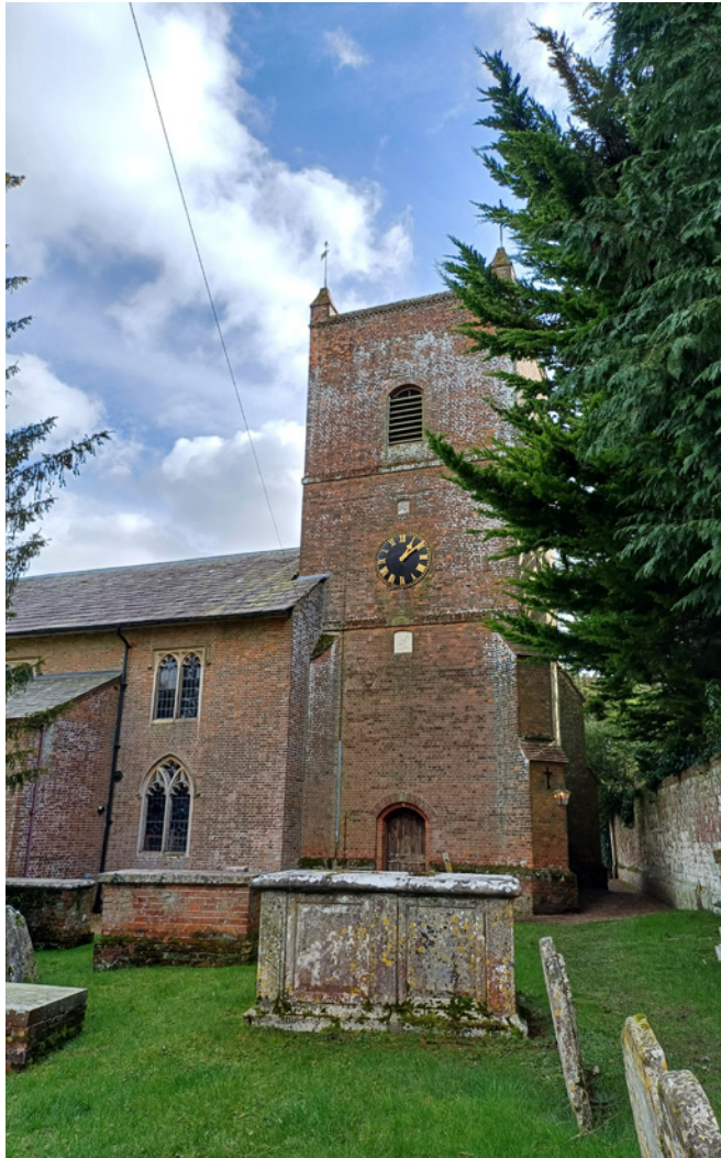
Heavy efflorescence (salt staining) across the brickwork on the church tower, which is particularly vulnerable to repeated cycles of wetting and drying due to its exposed position.
