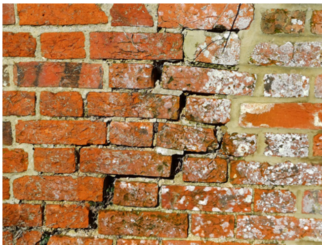
Lack of maintenance/repair to this section of boundary wall on Froyle Road has resulted in large open joints, which encourage water ingress and plant growth and can hasten the deterioration of built fabric.
