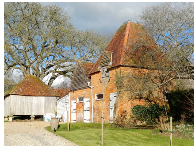
A stable block and hop kiln dating from the mid-19th century on the former site of Rockhouse Farm. Hop kilns, also known as oast houses, can be identified by their steeply pitched pyramidal or conical roofs. They were utilised to dry hops grown on the surrounding land. 10
