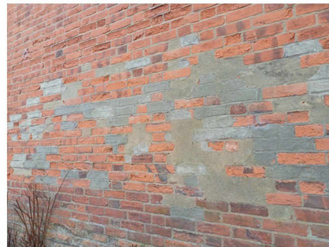
Large amounts of cementitious mortar have been applied to the wall of this historic building on Froyle Road. This will eventually have the effect of forcing moisture into surrounding historic bricks thereby causing further deterioration.
