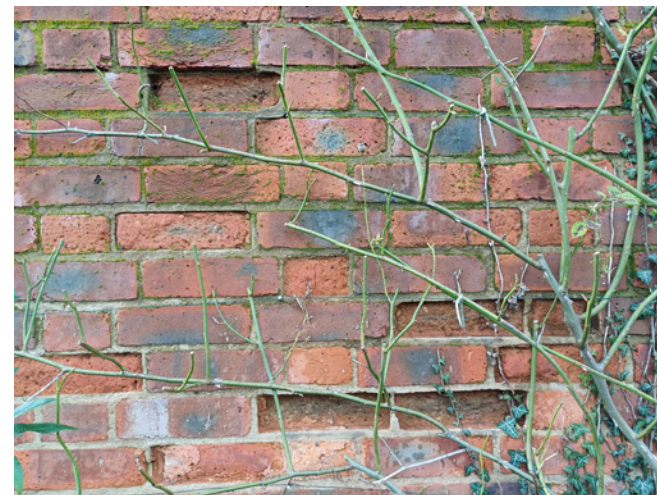
This photograph illustrates the damage caused to fabric through the use of cementitious mortar to re-point historic brickwork.
